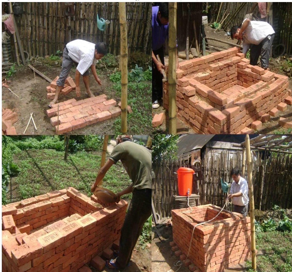
Figure 2. Different stages of construction of Zero Energy Cool Chamber (ZECC)
